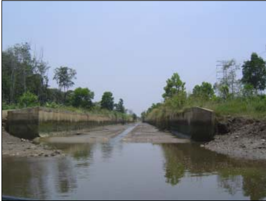
Photo E: View of the first drainage discharge outlet from the GIE.
