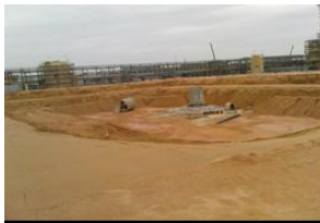
C3 – Flue-Gas Desulphurization (FGD)
