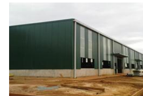
C6 – Production Storage
