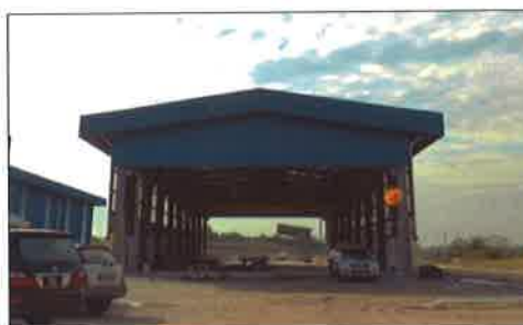
Tapak Projek Depoh Kempas Baru, Johor Bahru - Loco Shed (11.08.2014)
